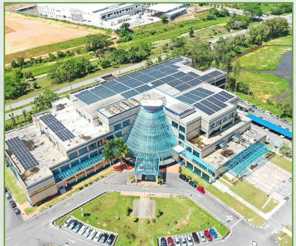
Solar PV Rooftop Installation in KHTP Business Centre
