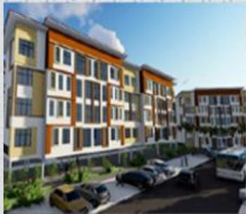
CENTRALIZED LABOR QUARTERS (CLQ)
