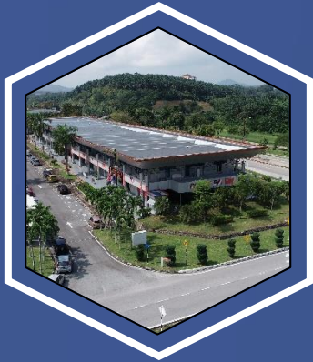
KHTP ADMINISTRATIVE CENTRE
