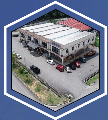
KULIM PERDANA SHOPHOUSE
